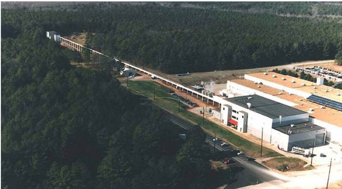
Figure 4: MSFC's X-Ray Calibration Facility (XRCF). The XRCF vacuum chamber (in lower right building) is large enough to hold any orbiter payload and sufficiently distant (530 m) from the sources (in upper left building) to produce the small source sizes ( < 0.2'' ) needed to test and calibrate Chandra 's sub-arcsecond x-ray optics.
